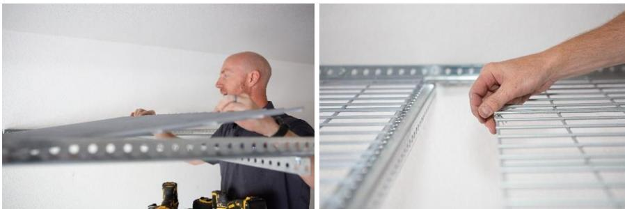
Place in the 2<sup>nd</sup> piece, pushing toward the first piece. Use 2 clips to bolt the edge of the 2nd deck piece to the bottom support. Use the provided ¼" nuts and bolts to secure the clips to the bottom support pieces. The safety clip should pass under the first deck piece and bolt to the bottom support. This 2<sup>nd</sup> decking piece will push against the first piece keeping it in place.
