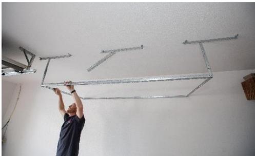
It is always recommended to leave the center support not connected until you have installed the decking material. Once your decking is installed you can connect the center support. Simply install the vertical post to the perimeter frame using the lock nuts and bolts provided. Use a level to ensure plum.
