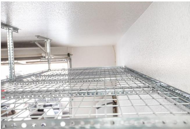
**The decking interior seams should all align with the bottom support pieces and should not be able to move side to side at all.**
