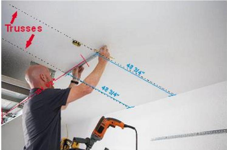
Using the 26" bracket as a stencil, mark the holes with a pencil where the trusses are located. Your vertical post must fall in between the two trusses and never outside of them. Set aside the 26" ceiling bracket.
