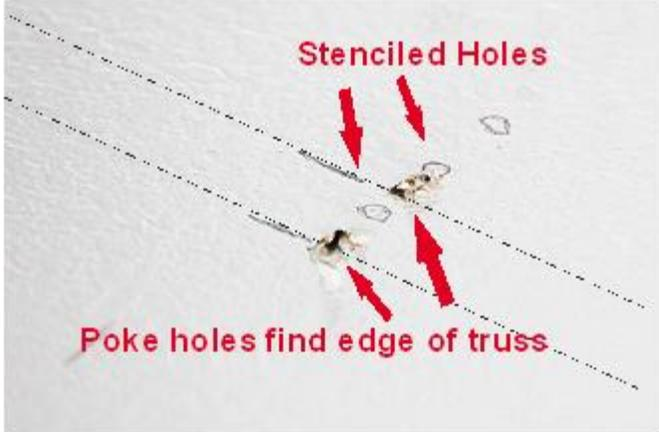
Pre drill the stenciled hole that is most centered with the wood beam with your 3/16" drill bit. You can slightly adjust this location to make sure you are drilling into the center of the truss.
