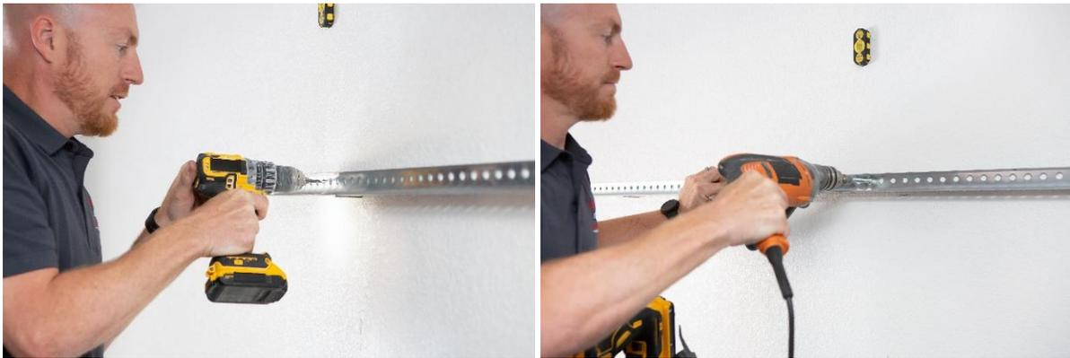
Wall mounted framing need a lag screw within 2ft of each end of the frame piece. This is minimum standard code for any wood framed wall.
