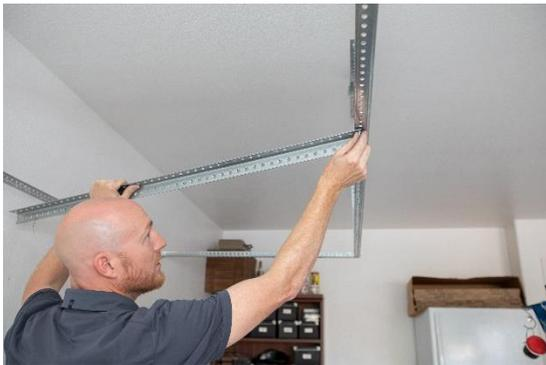
Then go back with a  $\frac{1}{2}$ " wrench and  $\frac{1}{2}$ " socket to tighten the rest of the way.
