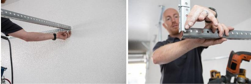
If you are connecting together multiple rack sections (example to create 4ft x 16ft unit) now is the time to connect the adjoining piece. (Shown Below) Butt the frame pieces together where you want to extend the next section. The 2 racks will share this vertical support and this will serve as the first corner of the next rack.
