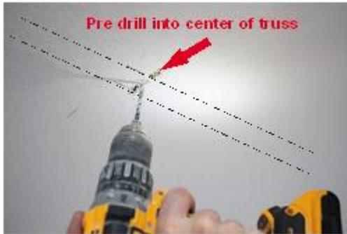
Mount the 26" ceiling bracket with the Lag bolts included using the predrilled hole.
